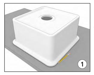
Temporarily place the product on the underside of the countertop. Mark outer edges on mounting surface.
